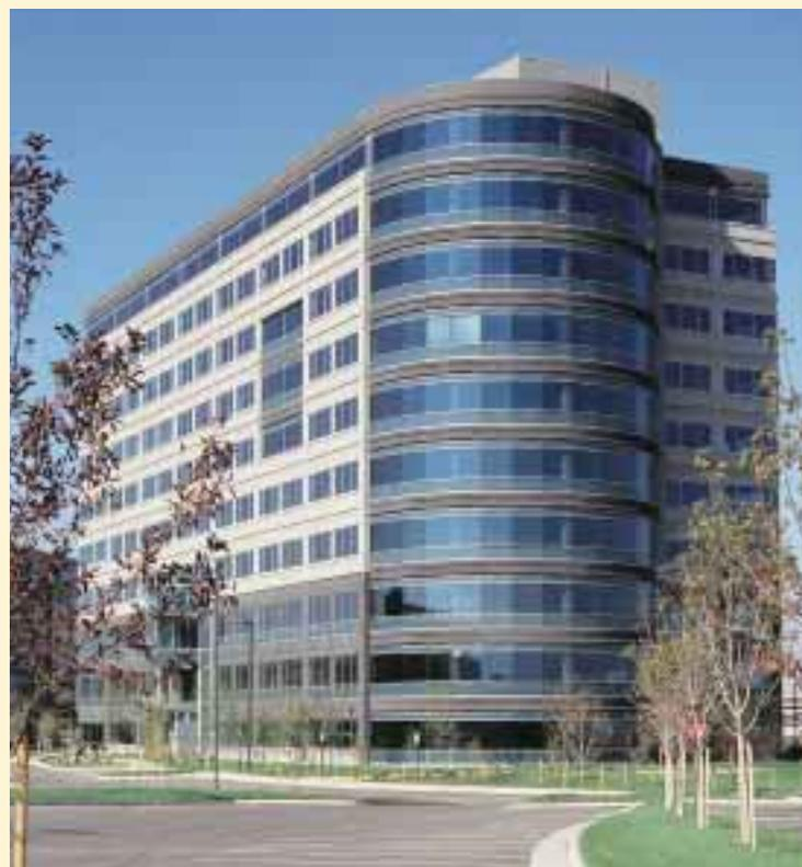
not only as the cladding but also as part of the structural system in supporting the precast floors. This provided large areas of glass because beams could be very thin, taking up a
