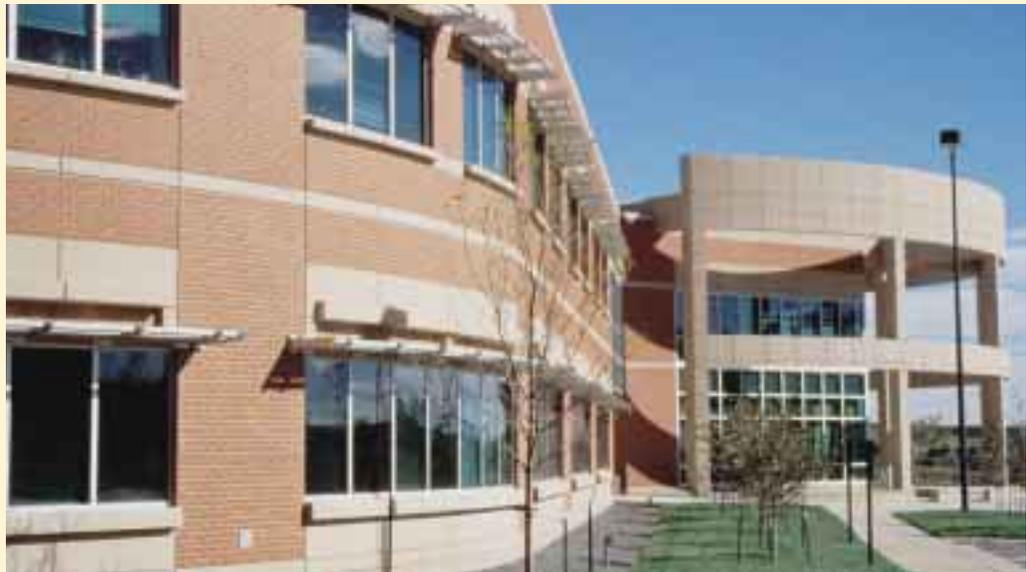
The Jefferson County District Attorney's Office Building, completed in 1997, uses a variety of precast concrete details and brick panels in the two-story, 52,000-square-foot structure. The design features a sweeping radius that is found on two corners of the building.
