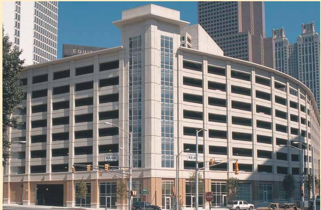
Cooper Carry has recently completed two parking facilities in Atlanta using architectural precast concrete as the primary building material. The Coca-Cola Parking Facility, an 825-car, five-story deck located at the company's headquarter complex, is constructed of precast concrete panels on a cast-in-place concrete structure. The SunTrust Parking Deck, a 750-car, eight-level parking facility located on an urban site, used architectural precast panels, textured-coated concrete and brick.
