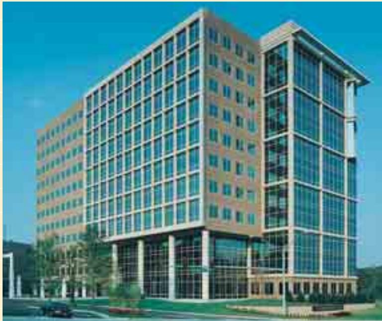
*Fig. 10: Solid precast vertical pieces are used on the Glenridge Highlands One project in Atlanta to define the corners and the transitions from curtain wall to precast at the corners. Originally planned as returns and channel spandrel covers, they were cast solid at the precaster's suggestion for economy and detailing simplification.*
