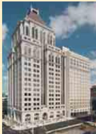
reveals in the vertical panels helped to modulate the precast panels to the scale of the original terra cotta blocks. (See Fig. 1 and 2.)
