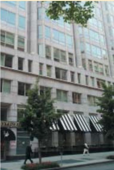
*This example of domestic pink marble stone clad precast panels and glass and metal clad high rise office building shows minor mineral fading which has occurred since the building was constructed in 1989.*
