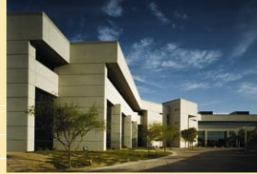
Fig. 9 – Cantilevered floor used to shade windows.
