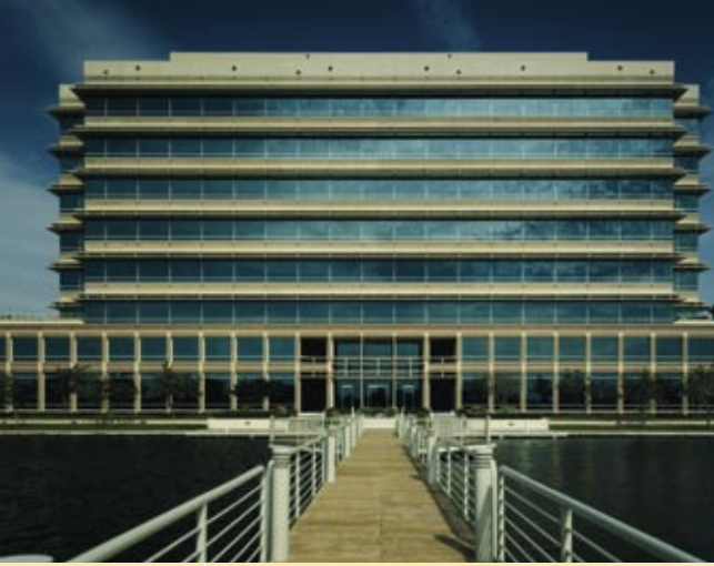
Fig. 2 – Horizontal sunscreen. Photo: © Brian Gassel/TVS & Assoc.
