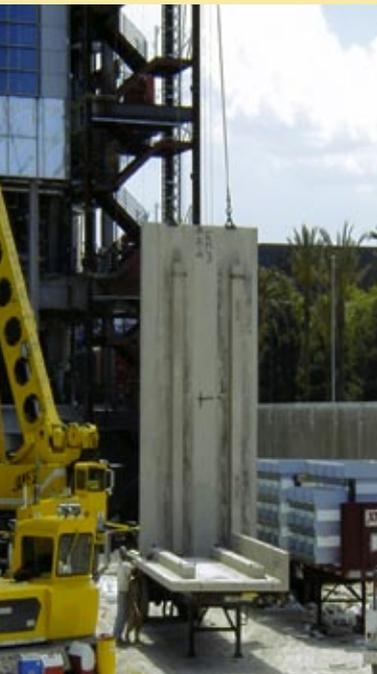
**Fig. 8 – The 6 in. thick x 22 ft. tall panels were reinforced with ribs spaced 6 ft. apart.**
