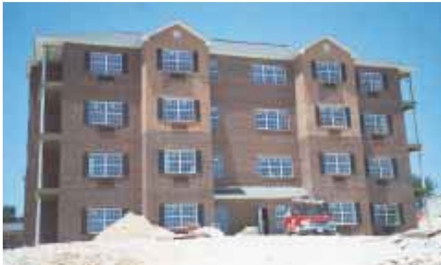
The Homewood Residence's 50 studio apartments feature hollowcore floor/ceiling units, which saved time and cost for the Westover Hills, Texas, project. The plank features a 2-inch layer of concrete on the flooring side and an acoustic spray and paint on the ceiling side.
