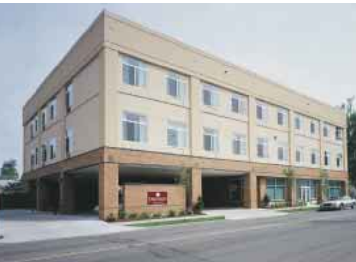
Morse Bros. Inc. Prestressed Concrete Group erected the precast frame on Emerson House, including beams, columns and hollowcore floor and roof slabs, in just 12 days. Photo: Bob Pool Photography
