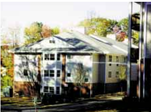
The new residence hall at Dominican College in upstate New York provides students with a living, as well as a learning environment. Precast concrete hollowcore plank provided quick erection time and fire-resistant flooring.
