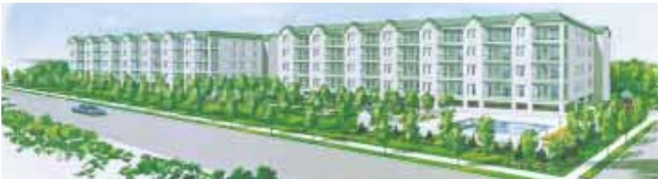
The Diamond View condominiums in Wildwood Crest, N.J., feature cantilevered balconies and walkways made of hollowcore plank, which also serves as flooring and ceiling elements. The second of the two 28-unit buildings will begin construction in September. Photo: ©Martin Photography
