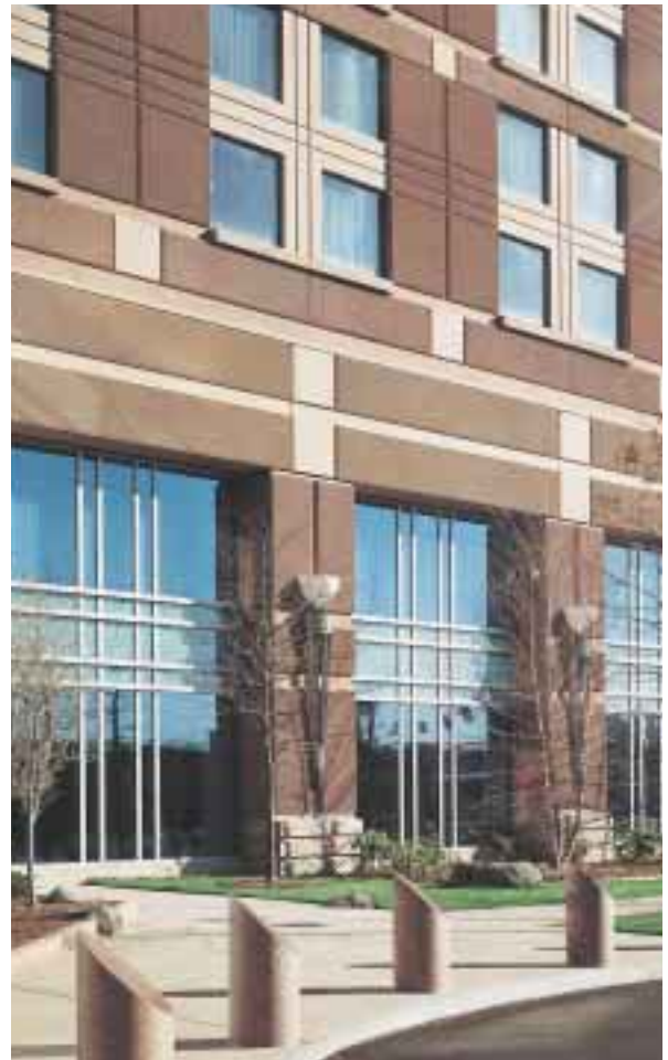
The precast panels were designed to reflect the module of the hotel rooms and the building's structural system. Individual panels contain both ribbed and smooth sections and two colors. Photos: ©Steve Rosenthal
