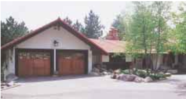
Precast concrete hollowcore plank were used to span the garage floor at this rustic home in Minnesota, creating a column-free room beneath, where the family installed an in-ground pool.
